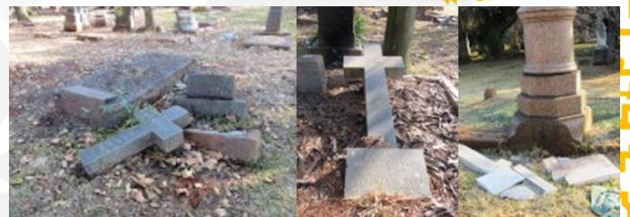
Image: Dilapidated headstone structures at the Brixton Cemetery
